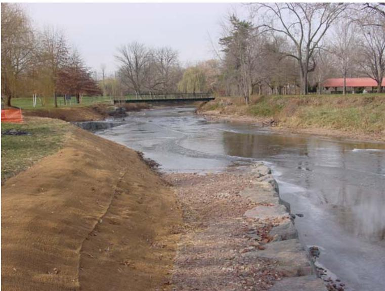
*Photo point depicting site after implementation of restoration project that included re-grading and the installation of coir matting and rock vanes. Note footbridge and pavilion in background.*
