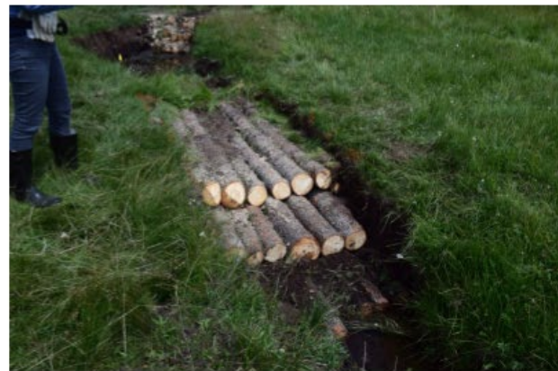
Log and Fabric Step Fall (K. Menetrey 2014)
