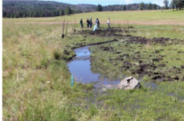
Hand-dug worm ditch (K. Menetrey 2015)
