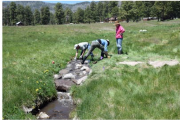
A volunteer crew with Albuquerque Wildlife Federation constructs a Rock Mulch Rundown (K. Menetrey 2019)
