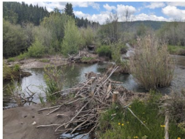
PALS that has accumulated woody debris after several years. Note sandbar development and side channel pool habitat forming downstream (P. Watson 2023)
